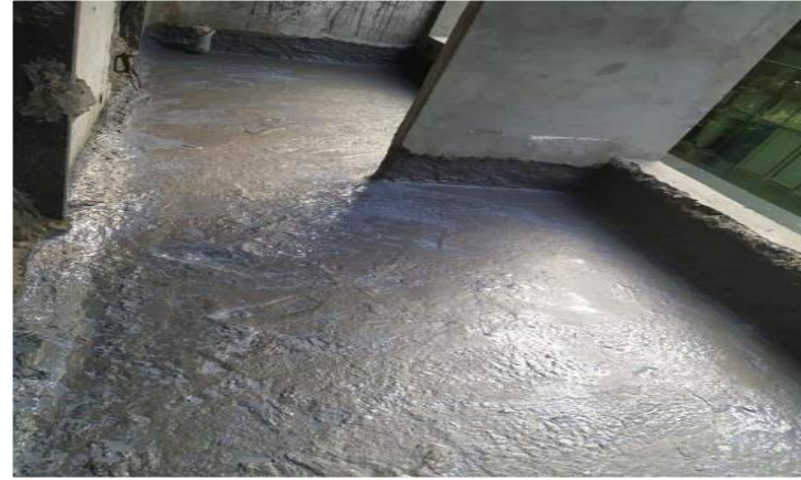
CEMENT BASE COATING
