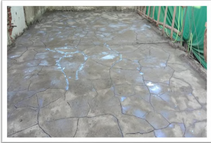
CRACK FILLING
