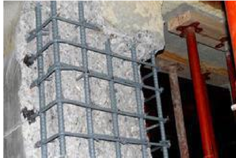
COLUMN BEAM REPAIRING
